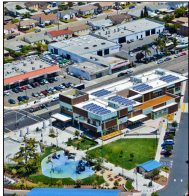
REACH Ashland Youth Center in the Ashland District, Aerial View, Image Courtesy of RossDrulisCusenbery Architecture, Inc.
