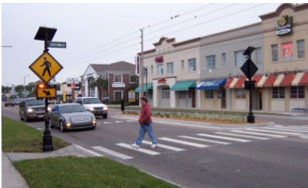
Pedestrian Activated Rectangular Rapid Flash Beacons (RRFB)s Can be Installed at Crosswalks to Increase the Number of Drivers Yielding for Pedestrians and Reduce Pedestrian-Vehicle Conflicts.
