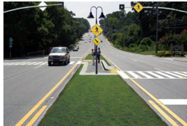
Example of how a Landscaped Median can Reduce Crossing Distance and Improve the Appearance of the Streetscape.
