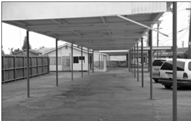
Existing West Eden Corridor Vacancies Contribute to an Incomplete Streetscape
