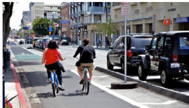
Example of a Protected (Class IV) Bikeway adjacent to On Street Parking, separated by painting strip and curb.
