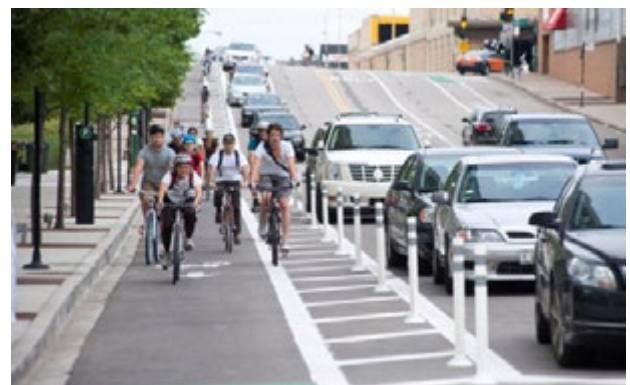
Example of a Protected (Class IV) Bikeway adjacent to On Street Parking, separated by temporary posts.
